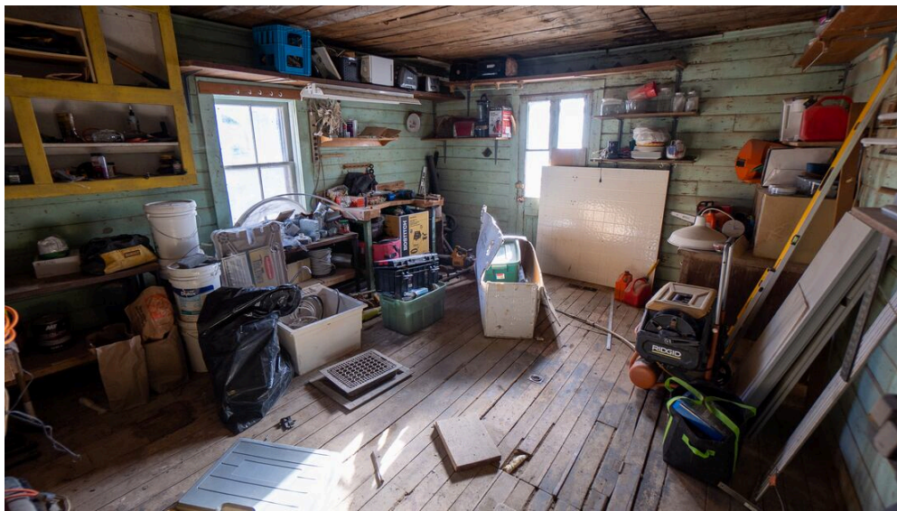
This room, currently used to store tools while the house is being renovated, will become the centre's new classroom. (Francis Ferland/CBC)
